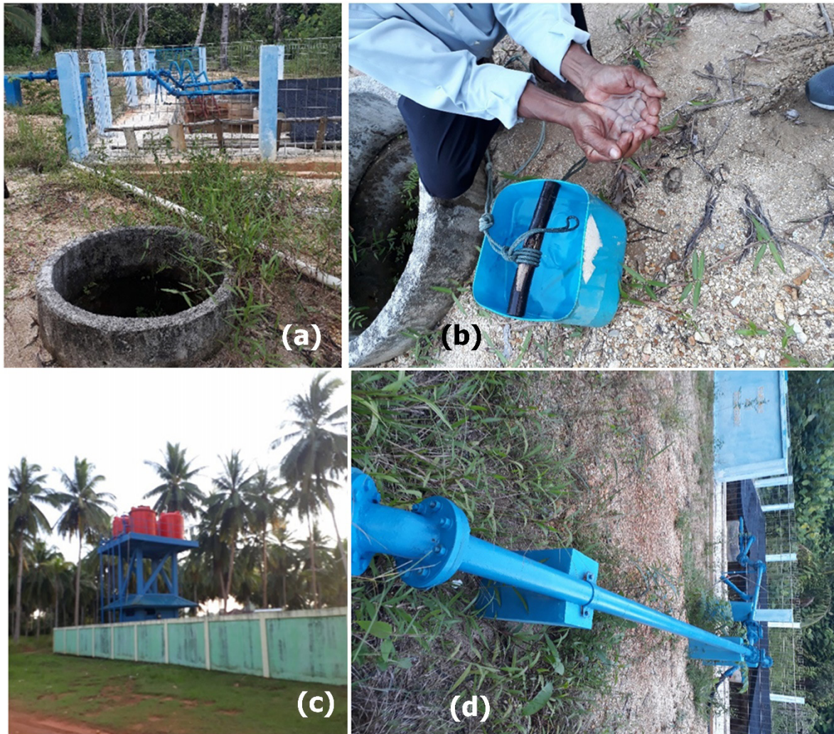
Figure 5. The Pamsimas facilities. (a) Pamsimas water well in Berakit Village, (b) Pamsimas well water quality, (c) Pamsimas water container in Berakit Village, and (d) Pamsimas pipeline to container in Berakit Village.
