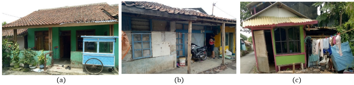
Figure 3. Housing Conditions in the Research Area: (a) Permanent; (b) Semi-permanent; (c) Non-permanent
