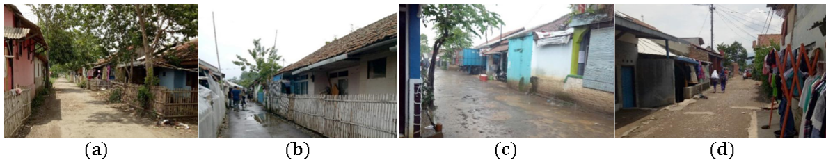
Figure 4. Conditions of Local Access Roads: (a) an asphalt road with potholes in Padaulun Village; (b) a narrow road in Padamulya Village; (c) a dirt road with puddles and mud after rain in Sukamaju Village; (d) a damaged road in Sukamaju Village
