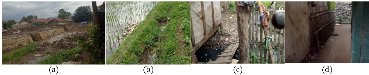
Figure 7. Components of the Drainage System in the Research Area: (a) Citarum, the estuary of the urban drainage system; (b) irrigation channels used to dispose of domestic waste; (c) stalled drainage channels; (d) flooding caused by lack of drainage.
