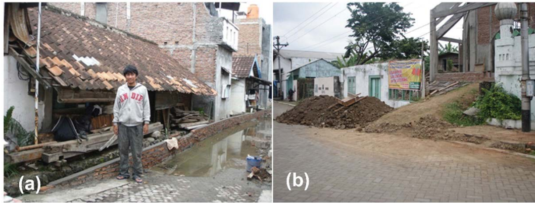
Figure 5. Adaptation efforts by elevating the road and building embankments around the house (a), elevating the house by landfill material (b).
