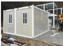
Gambar 14. Unit pabrikasi tipe kontainer (sumber: China Construction Third Engineering Bureau CO.,LTD., 2020)
