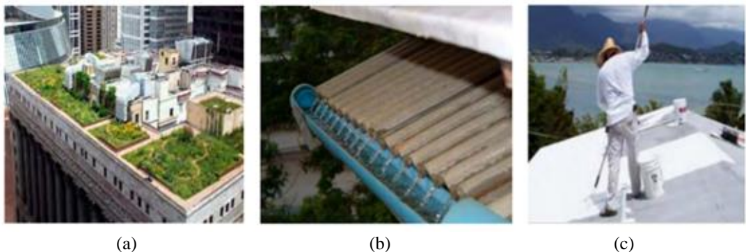
Figure 7. Type of roofs as a medium for implementing green roofs: green roof Chicago's city hall building in the US (a), roof pond Chiang Mai University located in Chiang Mai province (b), reflective white roof (c)
