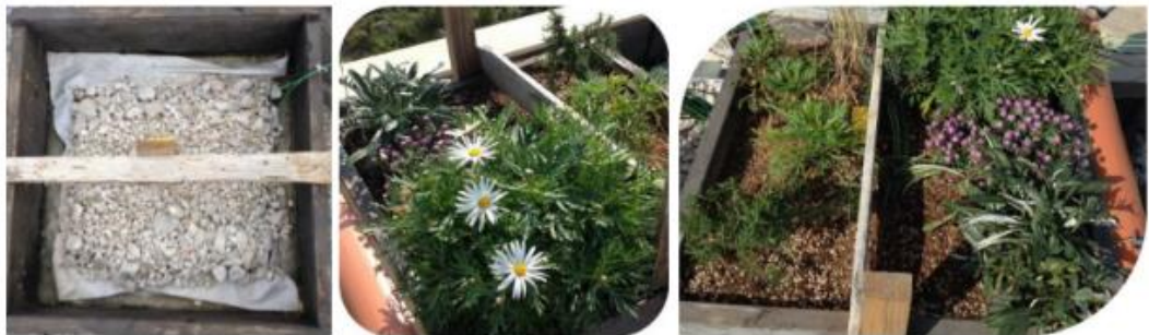
Figure 6. Green roof planting media that combine with rocks [20]
