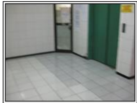
Gambar 19. Kondisi lobby lift RS. Moewardi Sumber: Survey Lapangan, 2009
