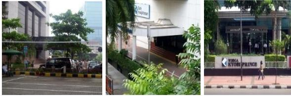
**Gambar 12.** Kanopi struktur beton atap polycarbonate; skylight
