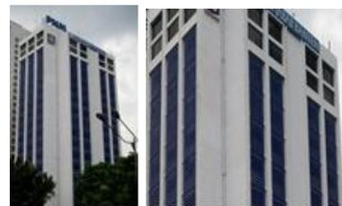
**Gambar 8.** Sirip-sirip semipermanen Wisma Arthaloka
